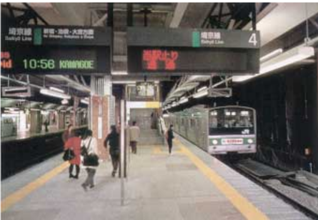
Saikyō Line Shinjuku - Ebisu Extension (JR East) To alleviate the overcrowded condition of the Yamanote Line during rush hours, the Saikyō Line connecting Omiya Station in Saitama Prefecture and Tokyo's Shinjuku Station added a 5-km extension to provide train services to Ebisu Station starting 16 March. Seventy-eight of the 187 trains to or from Shinjuku extend services to Ebisu, shortening the commuting time between Ikebukuro and Shibuya by 5 minutes and also greatly ameliorating the congestion between Shinjuku and Shibuya stations.
