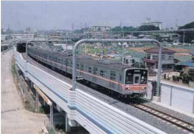
Toyo Kosoku Tetsudo Line (Toyo Rapid Railway) The Toyo Kosoku Tetsudo Line, covering a distance of 16.2 kilometers, started operations on 27 April between Nishi Funabashi and Higashi Katsutadai stations. The new Toyo Rapid Railway and Teito Rapid Transit Authority's Tozai subway line offer 166 direct train services on weekdays and 134 on weekends, and the commuting time between Higashi Katsutadai and Otemachi stations is now reduced to about 46 minutes.
