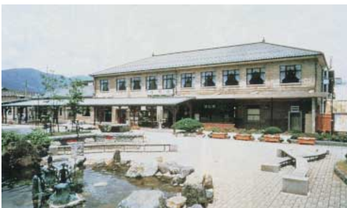
Hotel 'Folkloro' Tono (JR East) The old Tono Railway Station in Iwate Prefecture, 500 km north of Tokyo, doubles as a rural railway station and pleasant country hotel. Tono is a popular tourist destination symbolizing the traditional virtues and pleasant lifestyles of regional towns. It is a reasonably-priced Bed & Breakfast type hotel.
