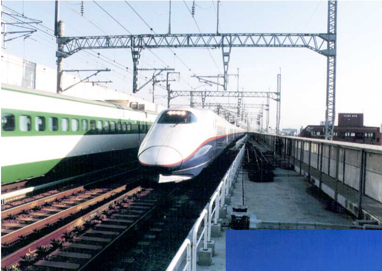
Newly-built E2 EMU on test run near Takasaki (Japan Railway Construction Public Corporation)
