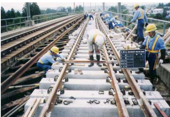
Laying mixed-gauge track
