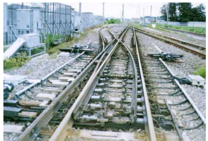
Mixed-gauge switching point
