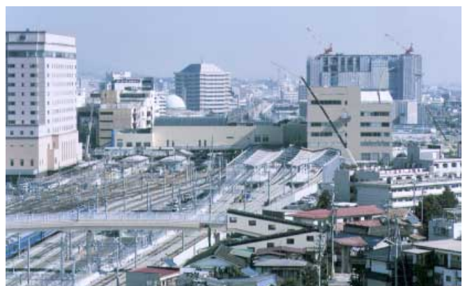
View of Nagano Station with new shinkansen platforms
