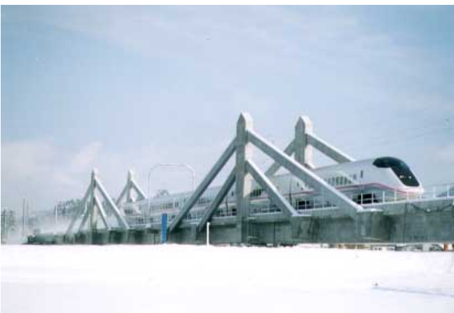
E3 test-run train crossing Tama River near Kakunodate on Tazawako Line (JR East)
