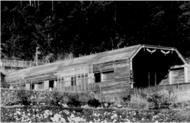
This hood at the entrance to Ohirayama Tunnel (6640m) on the San'yo Shinkansen is 49 meters long. If it had been constructed at the same time as the line, it would have been concrete. (JR West)
