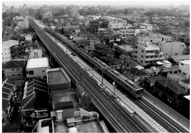
Construction site of quadruple track near Soshigaya-okura Station (Odakyu Electric Railway)
