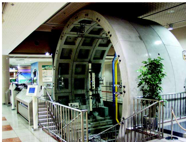
Three concrete tunnel segments with various trackside equipment
