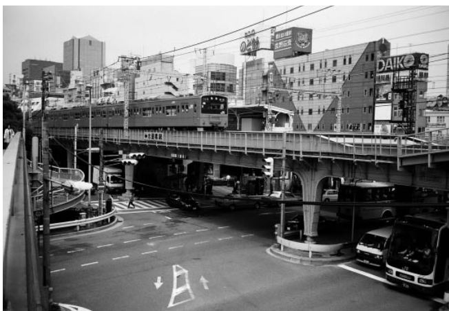
Suidobashi viaduct (1931) over Hakusan Street
