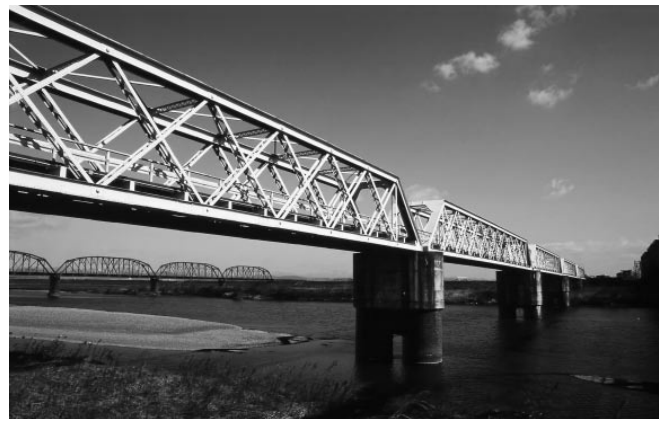
Ibigawa Road Bridge (1887) converted from Tokaido Main Line Railway Bridge (Author)
