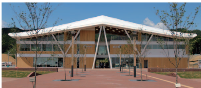
Rebuilt Onagawa Station (Onagawa Town)
