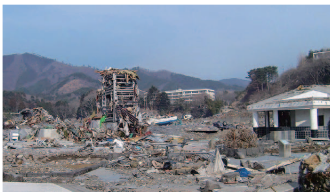
Old Onagawa Station after tsunami. Only the elevator shaft (centre) and rest room (white building, right) remained standing (Onagawa Town)
